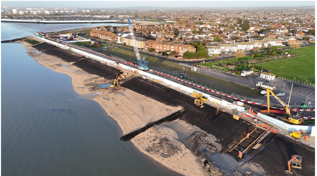
Works on the revetment at Thorney Bay and Labworth Cafe
