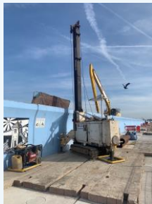
Piling rig at Fisherman's Corner
