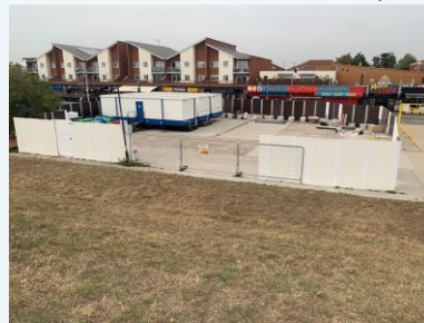
Satellite compound 2 set-up
